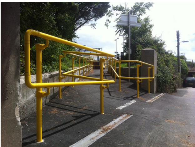
Fig. 2 Replacement of the crossing with the new access has significantly helped to improve the safety in the area
