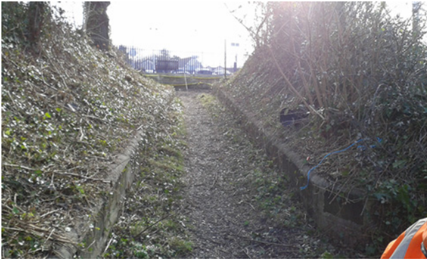
Fig. 1 Replacement of the crossing with the new access
